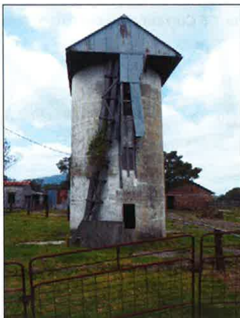
Figure 22: Concrete silo (structure J)
